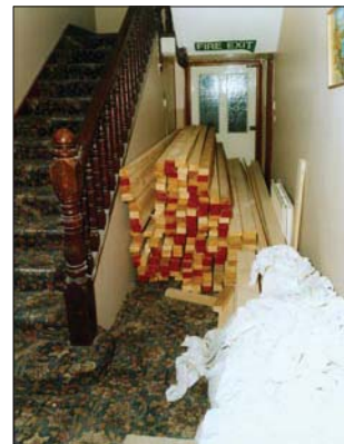
Figure 6: Picture of blocked corridor
